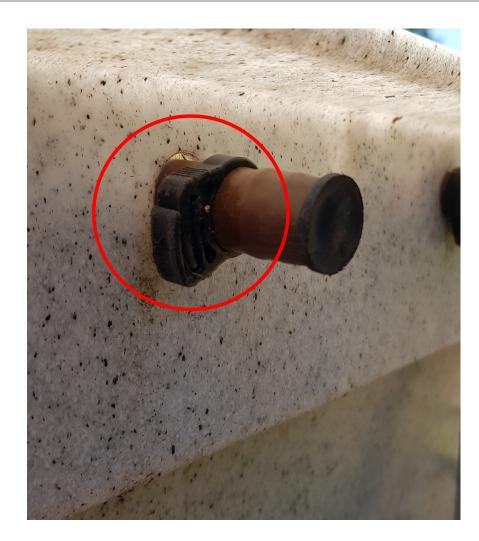
Finally, pull containers apart (taunting all irrigation lines). The ratchet clamp should now be 'flush' with your containers.
